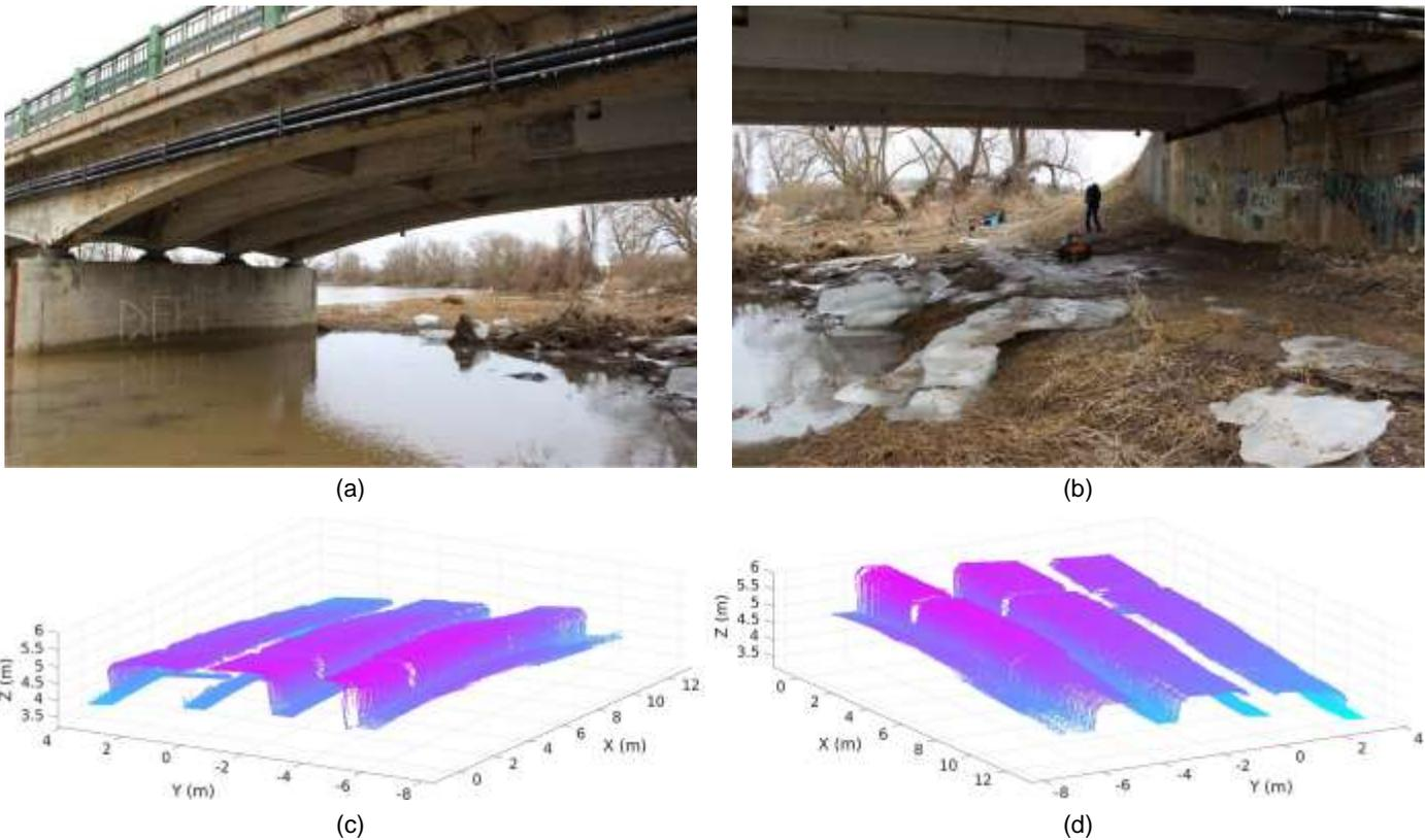
Fig. 9. Conestogo River bridge images and mapping results: (a) isometric view of bridge soffit, looking northeast (image by Nicholas Charron); (b) isometric view of bridge deck soffit, looking southeast (image by Nicholas Charron); (c) bridge soffit 3D map, looking north; and (d) bridge soffit 3D map, looking south.
