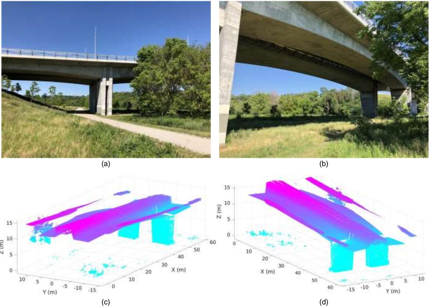
Fig. 10. Fairway Road bridge images and mapping results: (a) isometric view of bridge soffit, looking east (image by Nicholas Charron); (b) isometric view of bridge soffit, looking southeast (image by Nicholas Charron); (c) bridge soffit 3D map, looking southeast; and (d) bridge soffit 3D map, looking northeast.
